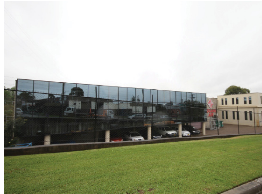
Figure 8: Atkinson Street view of the subject site, looking east
