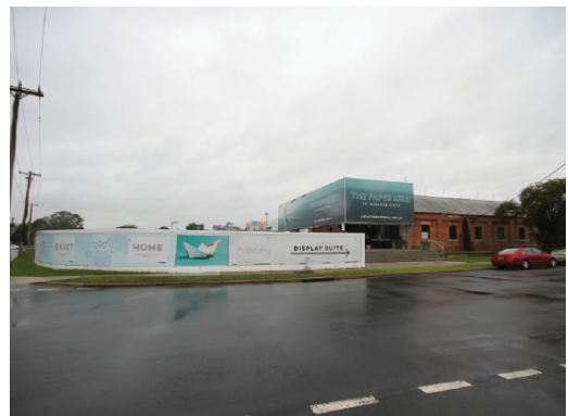
Figure 6: View from the corner of Atkinson and Shepherd Streets, showing the heritage listed McGrath Services Centre approved for adaptive reuse as a residential development
