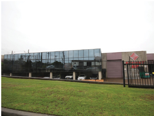
Figure 9: Atkinson Street view of the subject site
