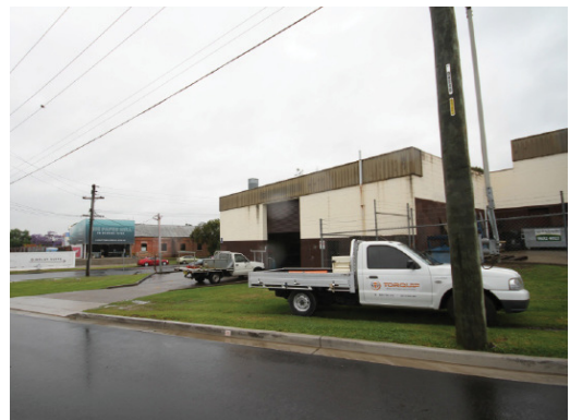
Figure 4: View along Atkinson Street, showing the light industrial building stock opposite the subject site
