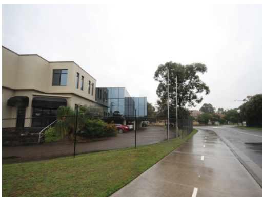
Figure 11: View looking north along Shepherd Street, showing the light industrial buildings on the subject site
