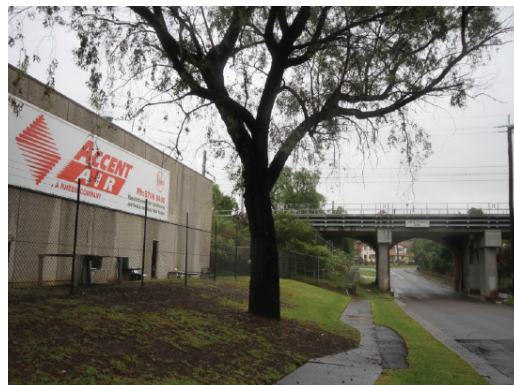
Figure 3: View looking west along Shepherd Street, showing the relationship between the heritage listed Railway Viaduct and the subject site
